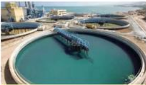
Ponds for water treatment
